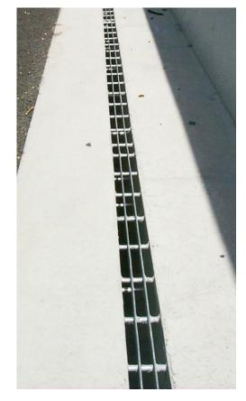
Figure 1 - SlimDrain Standard Trench Installation Detail
