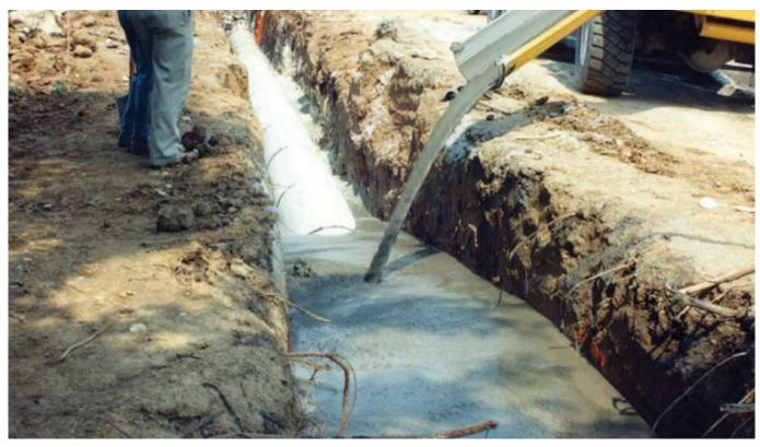
Figure 8 - Filling of service trench with flowable fill
